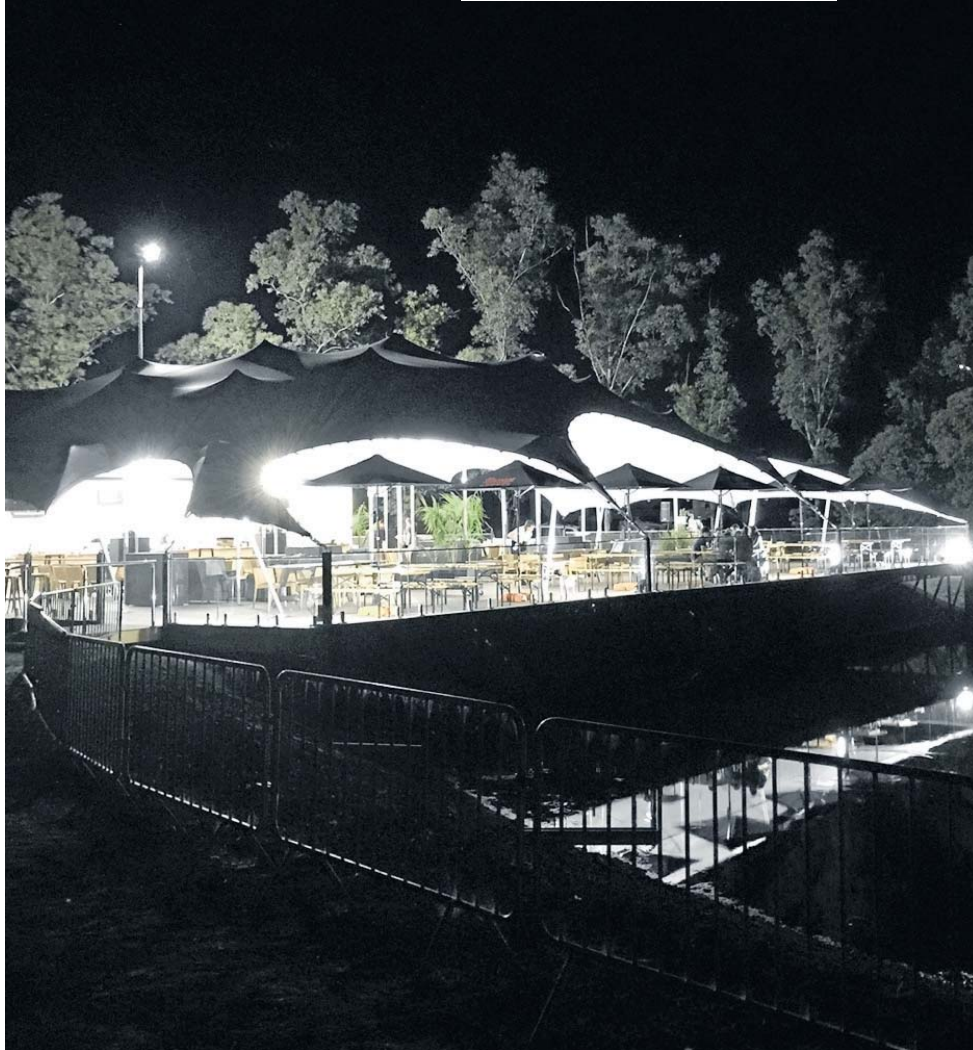
The Deck at Rochford Wines is a new food and entertainment area at the business. 163108 Picture: CONTRIBUTED
